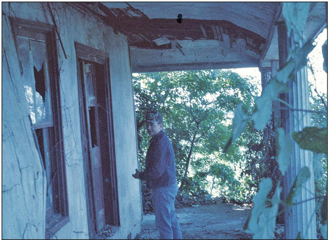
The house in Lyells where Menokin's woodwork was kept.
