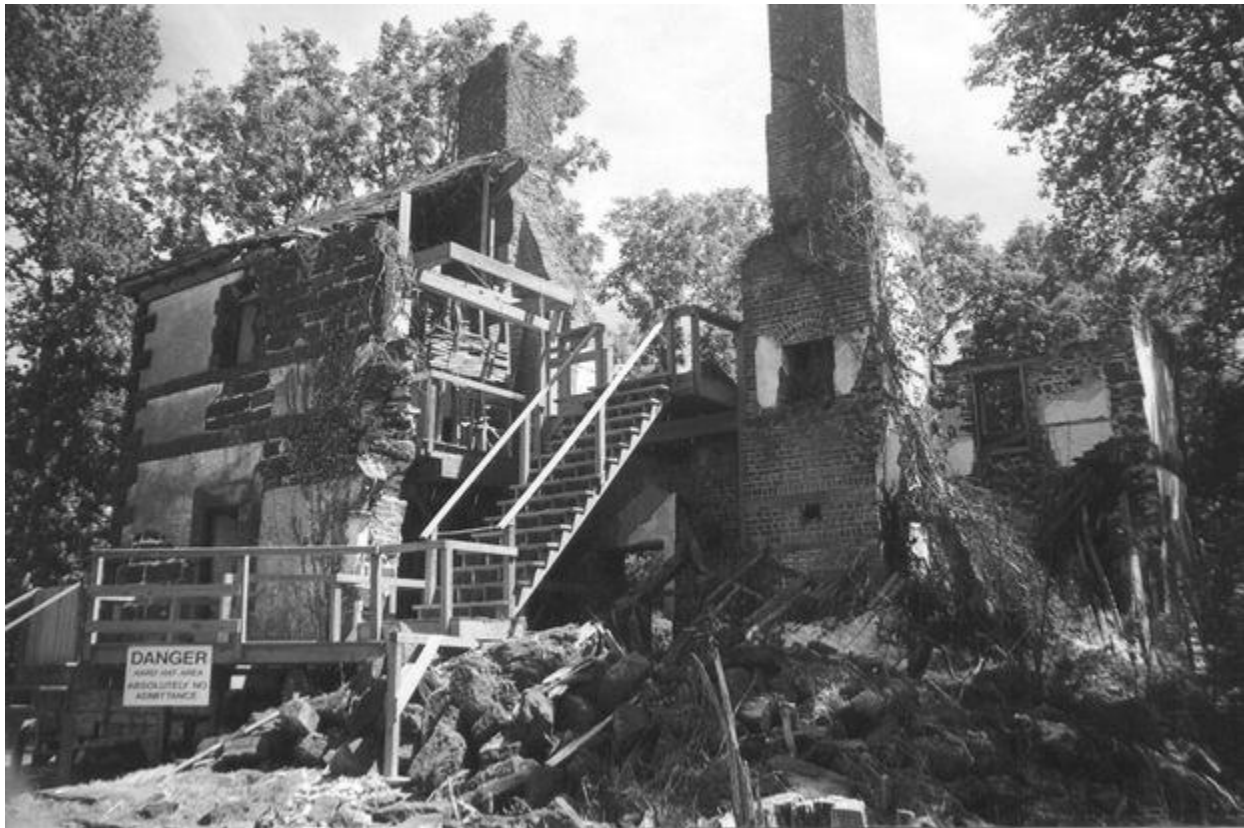
Historic image of Menokin, damaged by a falling tree PHOTO: MENOKIN FOUNDATION
