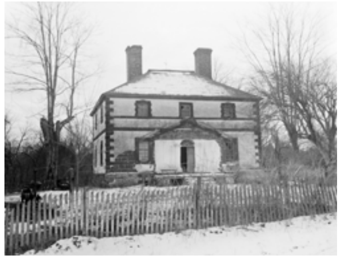
Menokin, north façade, 1940
