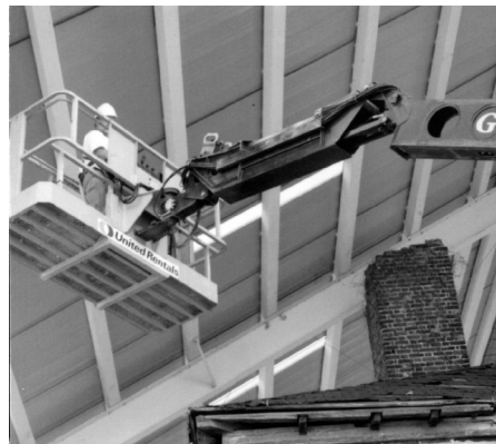
Laser scanning and the engineer's investigation were aided by a high-lift.
