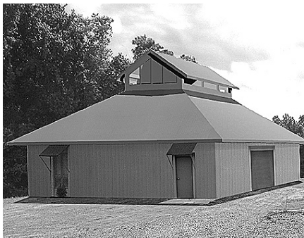
Image of the Menokin storage and assembly building
