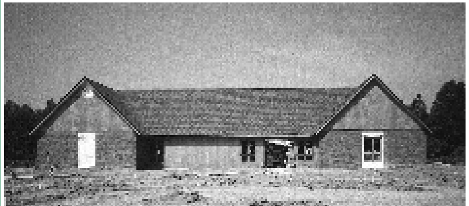
King Center construction under way
