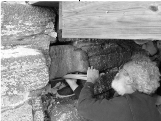
Masonry conservation work at Menokin, Spring 2007
