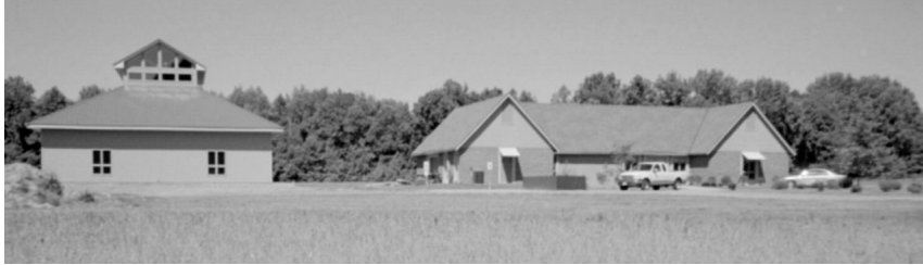
The new storage facility to the left of Visitors Center houses architectural elements excavated from the ruin.
