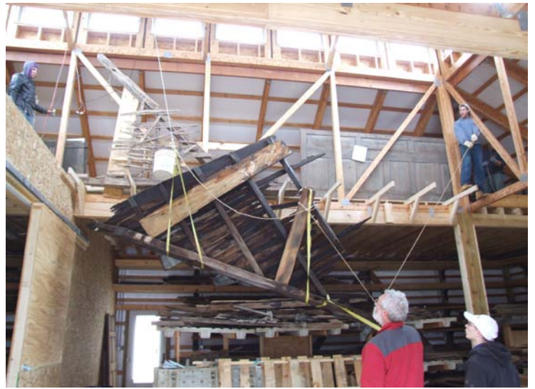
Moving assembly 2005-052 into the wood barn
