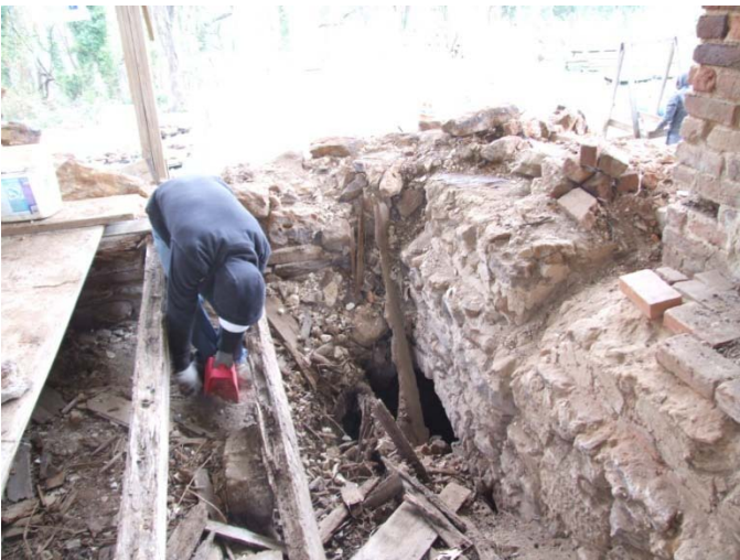
James cleaning out the South Chamber
