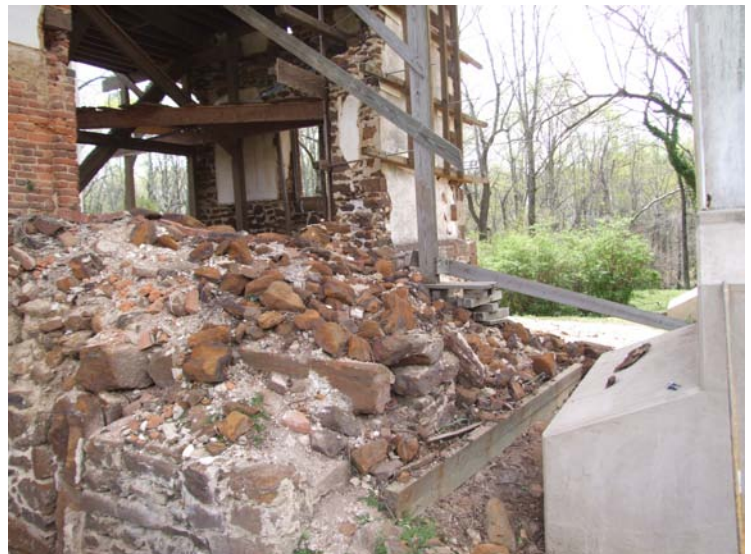
The Southwest Quadrant before excavation
