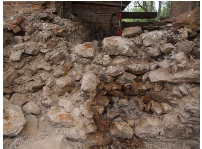
Visible Exterior West Wall!
