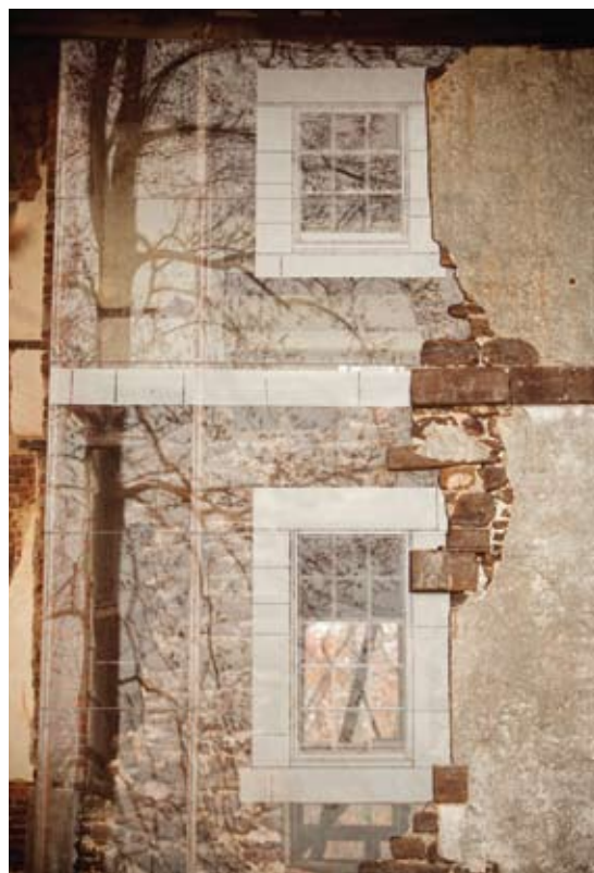
Above: architectural drawing of the north façade and photo from the 1940 Historic American Buildings Survey. Right: installed in 2009, a temporary acrylic wall protects the east interior and gives visitors a glimpse at how the glass walls will be structured.
