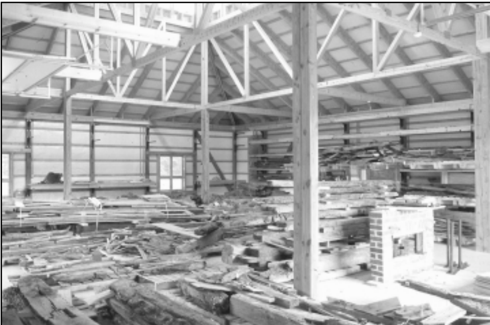
Interior of new Storage Building.
