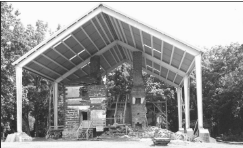
Menokin "under roof" with shelter and skylights.
